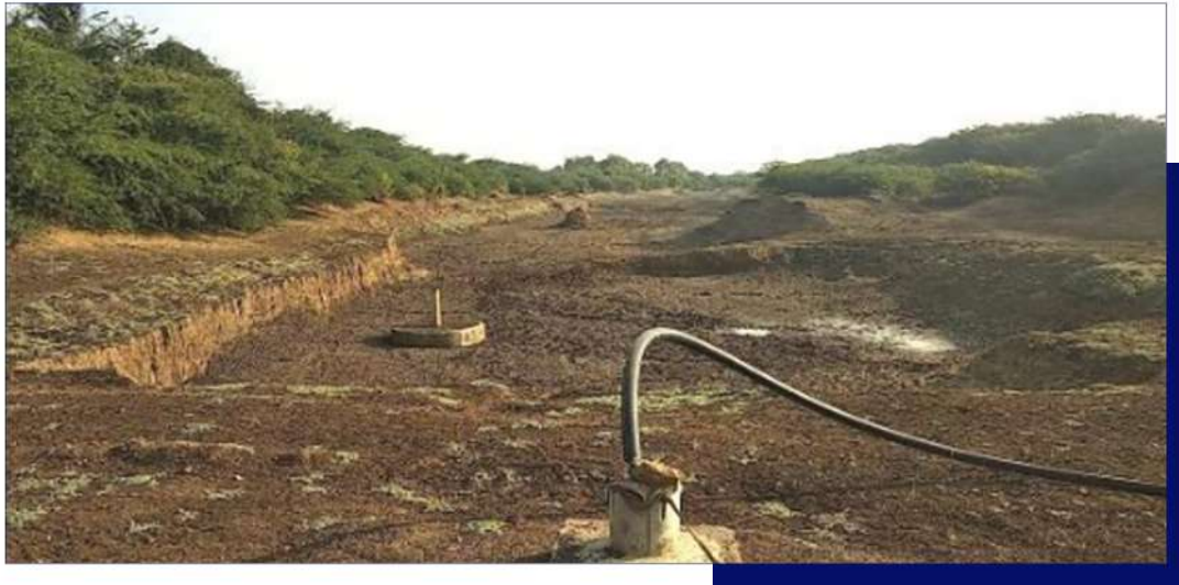
Figure 5. Overview of various structures developed under the intervention
