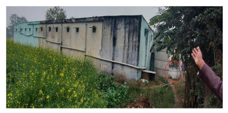
Collecting water from different roofs for diverting to dry-well (shown in red circle)
