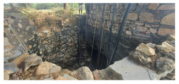
Well in the central part of the whole area is treated as withdrawal structure, with number of pumps for different zones
