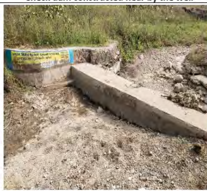
Check dam constructed near by the well
