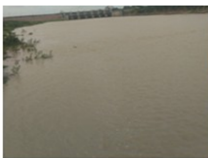
Barrage on Son River in Anuppur
